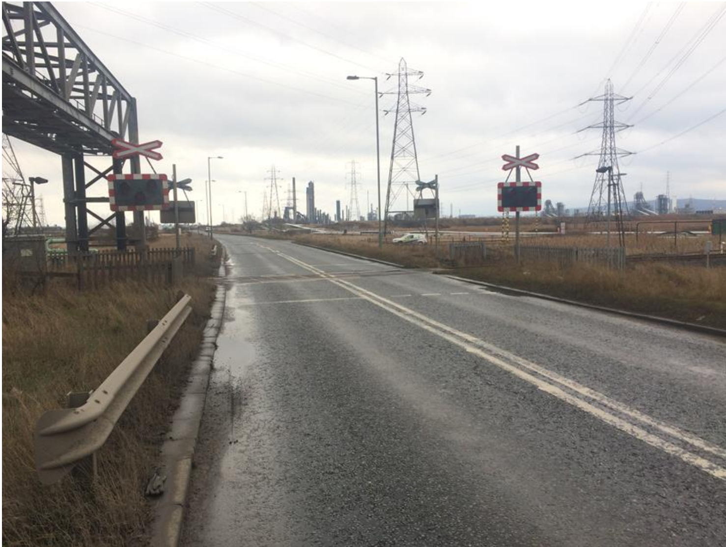
Station Road, Billingham
